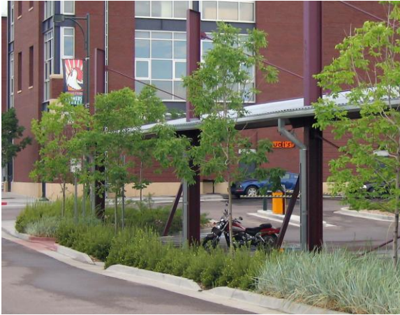
Figure 1 Rain garden in Stapleton Redevelopment, Denver, Colorado
