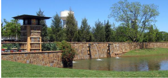
Figure 3-Detention pond in Colleyville, Texas
